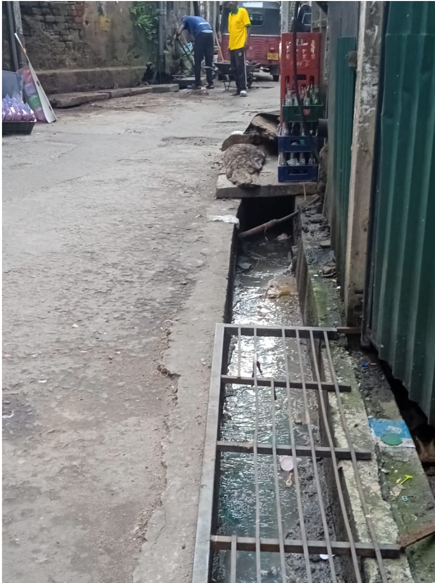
Figure 5: Clogged drains at Ali Mudukkuwa cause chaos during rainy days, underscoring the need for effective drainage management.
